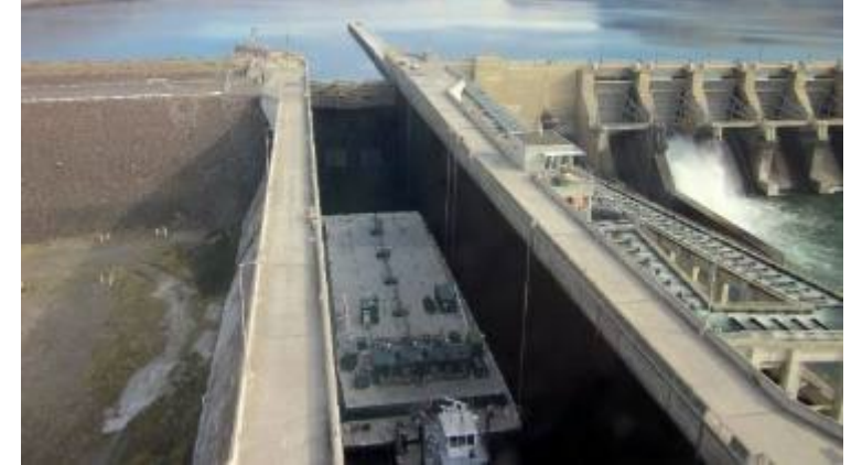
John Day Lock Length: 650 feet Max Lift: 113 feet (Highest in the Nation)
