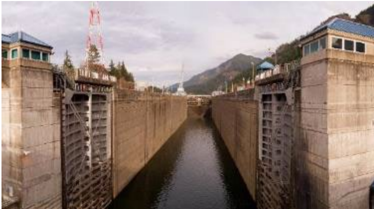
Bonneville Lock Length: 676 feet Max Lift: 90 feet
