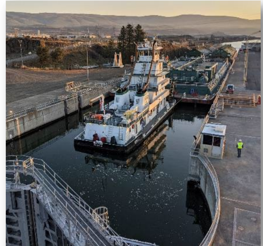
The Dalles Dam Navigation Lock
